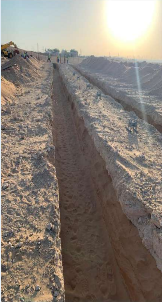
description: Trench clean
